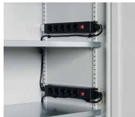
Side panel installation
